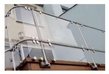
8mm Polycarbonate rounded at the corners. Q Railing Clips for 43mm bars gripping the plastic above and below, they should not be used on the sides. Q railing plug attached to the wood to hold the bottom panel (note this is designed to go through a hole in the plastic) Glass is too heavy to go on existing bars
